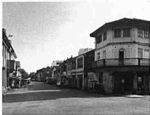
Shophouses in Penang. (Photo Cheang Yik On)
