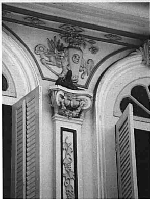
ABOVE: Detail of a terrace house façade in Malacca. Between the first floor windows a pseudo-Corinthian pilaster, with a ceramic figure on top, and moulded in plasterwork a relief showing a Greek vase, set against Chinese clouds and the lingzhi , the sacred fungus of immortality. (Photo H. Lin Ho)
